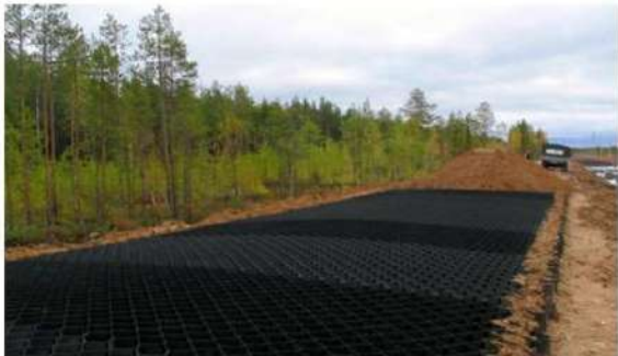
REINFORCEMENT OF WEAK BASES AND CONSTRUCTIVE LAYERS / ROADS
