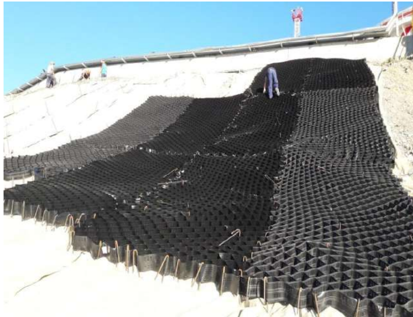
50m slope using traditional geocell
